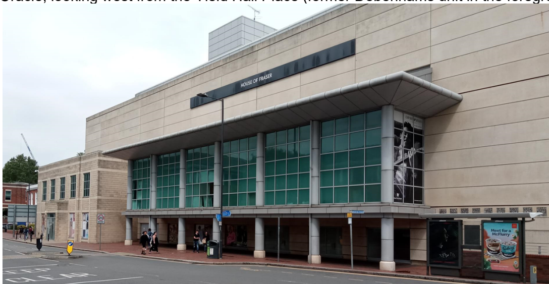
The Bridge Street elevation (unit occupied by House of Fraser).
